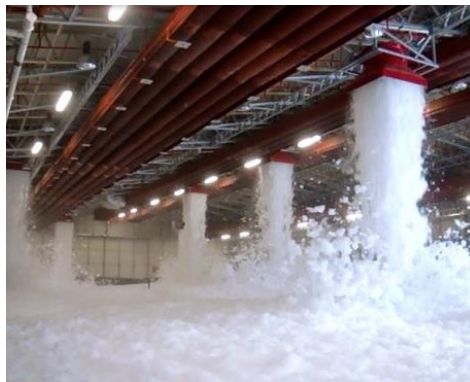
Figure 1 Foam sprinkler system [3]
