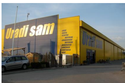
Figure 2 – Appearance of the building before the fire
