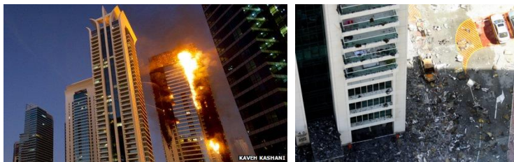
Figure 1 – Tamweel Tower blaze in Dubai (7)
