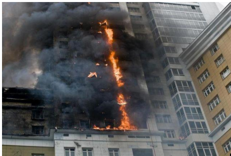
Figure 3 – Fire in a freshly constructed apartment building in Moscow [11]
