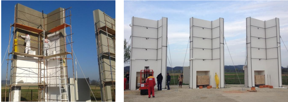
Figure 10 – Erecting the specimens (left), finished specimens (right)
