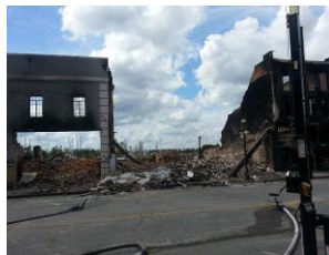
Figure 6 – Collapsed building after fire (13)
