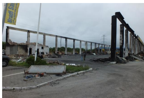
Figure 8 - Appearance of the building sight after the fire
