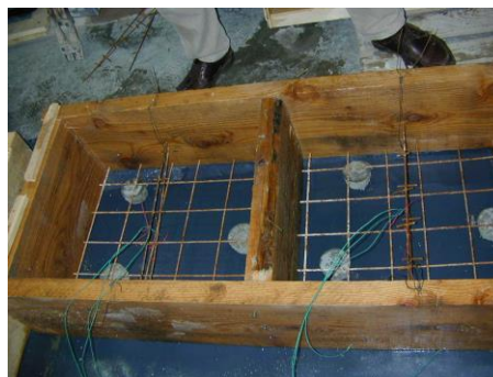
Figure 4 Placement of thermocouples before concrete casting
