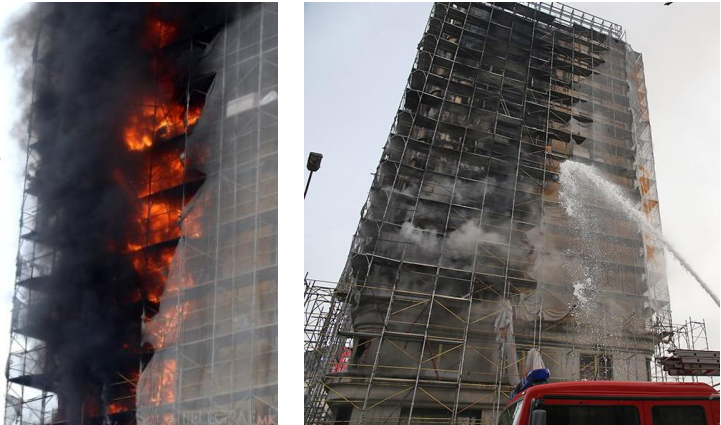
Figure 11. Toxic gases released from the burning façade made of EPS
