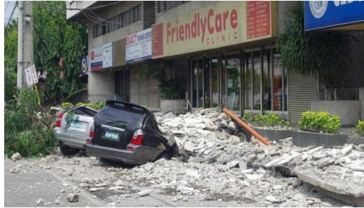
Fig. 33. Debris from a building fallen on a car
