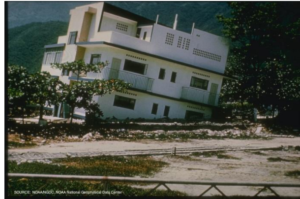
Fig.20b) Sinking and overturning of a building
