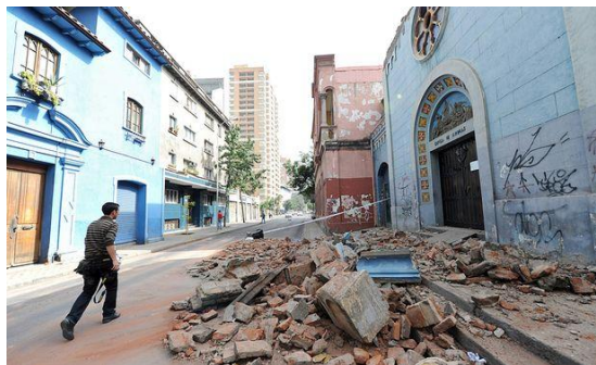
Fig. 26. Debris from a fallen facade
