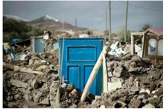
Fig. 16a) Almost all non-engineering structures collapse Fig.16b) Debris left from non-engineering structure
