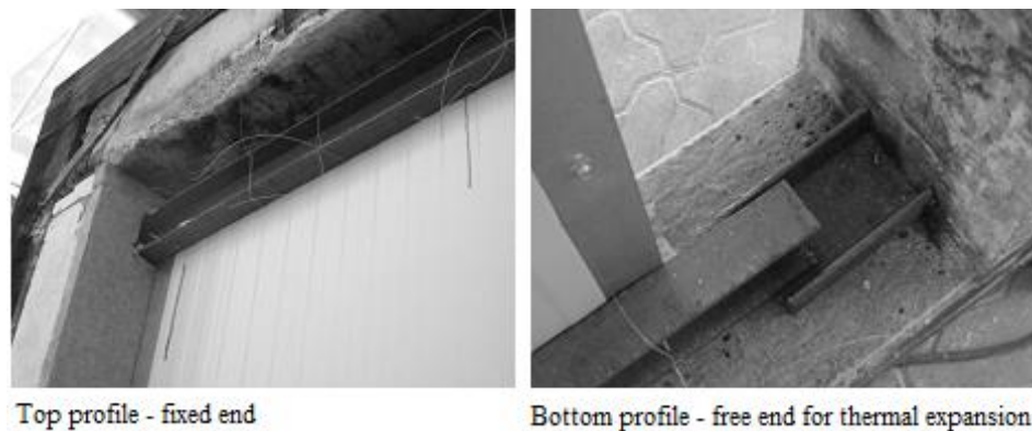
Figure 2 Panels were fixed to load-bearing steel profiles
