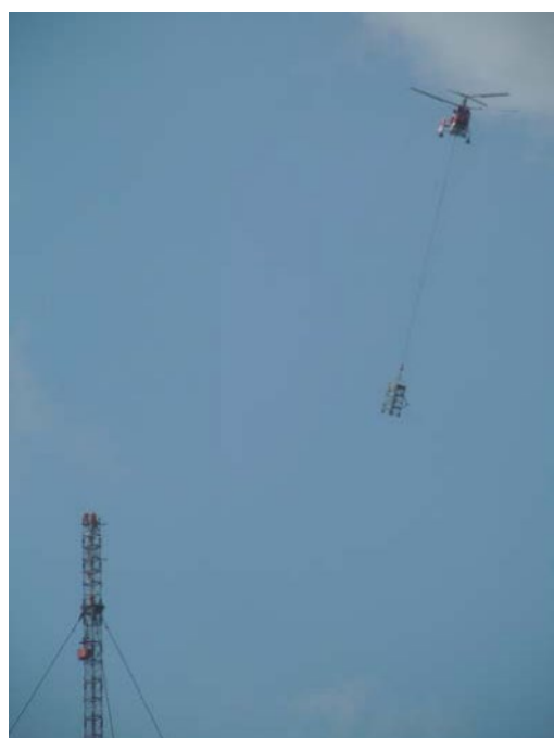
Figure 7. Helicopter in use
