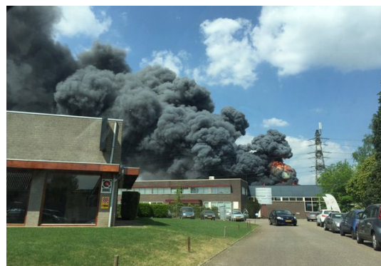
Figure 2. Fire in sports hall , Moergestel, Netherlands, 2016. [4]
