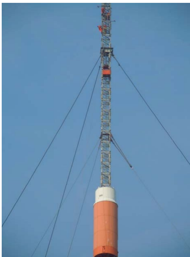
Figure 5. Temporary guy and elevator
