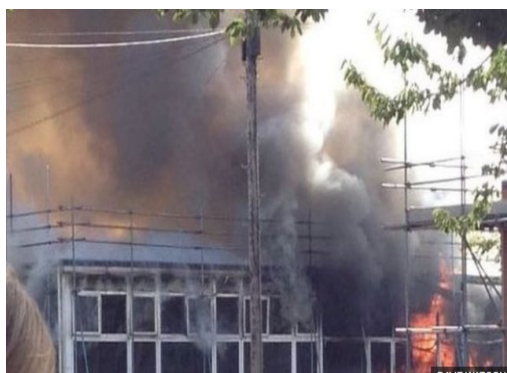
Figure 3. Fire in school hall-building in Normanton, Engleska, half of the building was on fire, 2015 [5]
