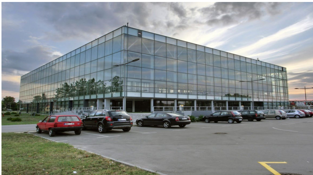
Figure 5. The appearance of the sports facility “Crystal Hall”
