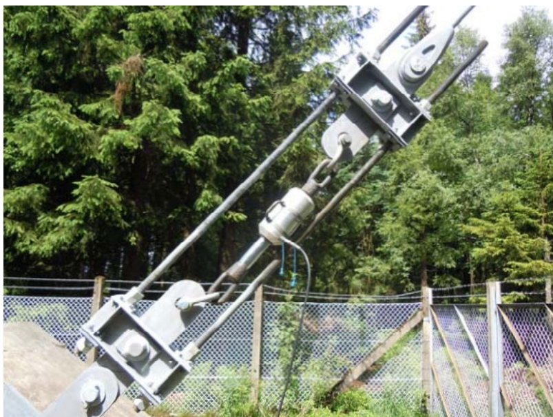
Figure 10. Pre-stressing of the cables
