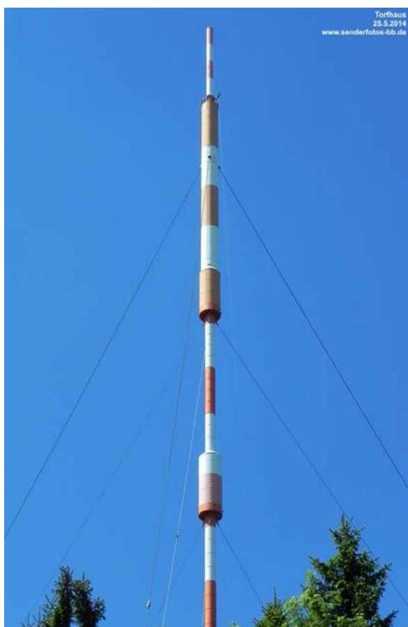
Figure 4. Mast in May 2014 [2]
