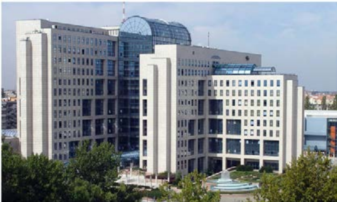
Figure 5 - The appearance of the NIS Business Center
