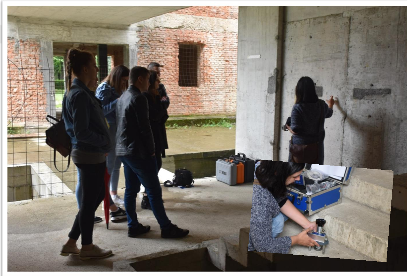
Pull off adhesion testing demonstration in existing concrete structure
