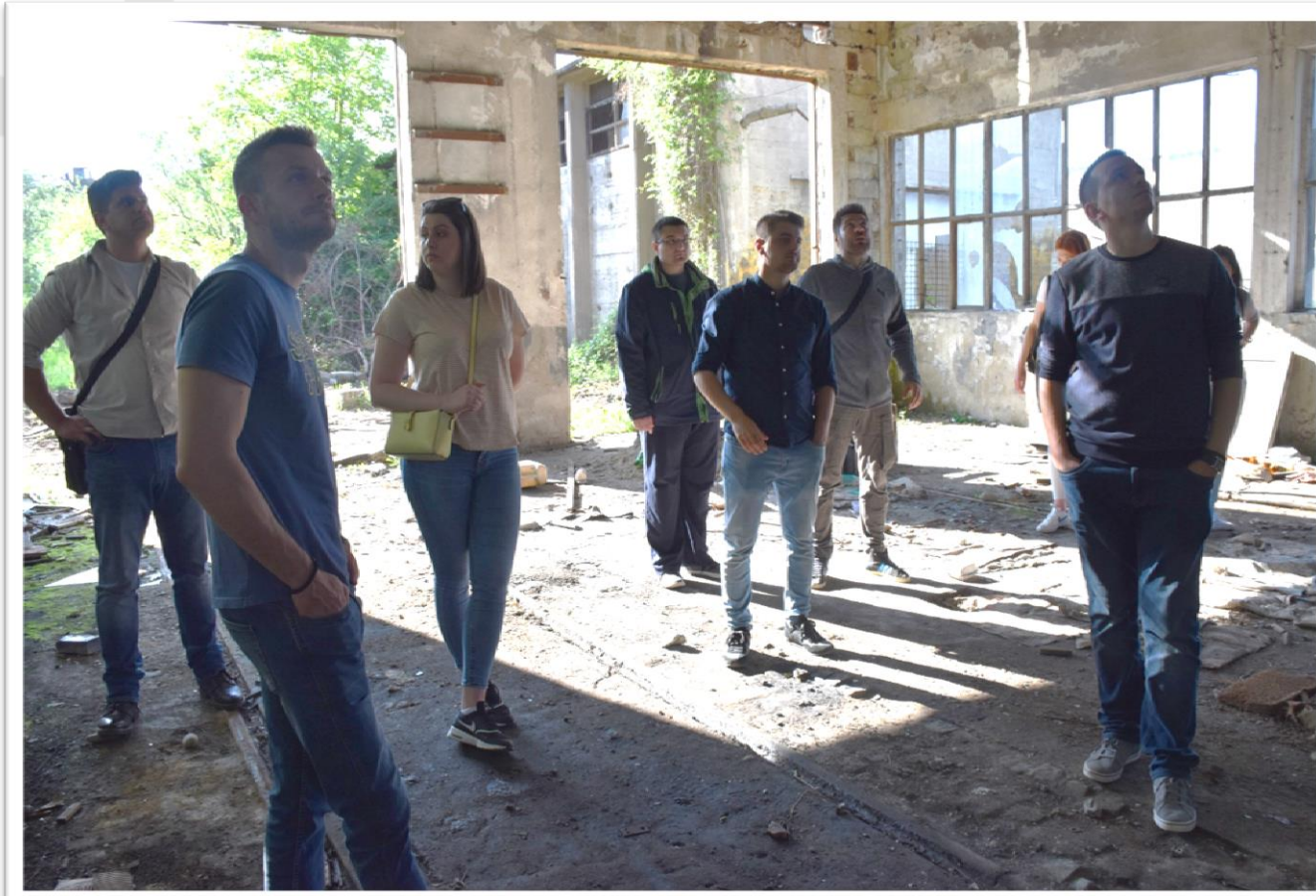
Assessment of Damaged Structures – site visits
