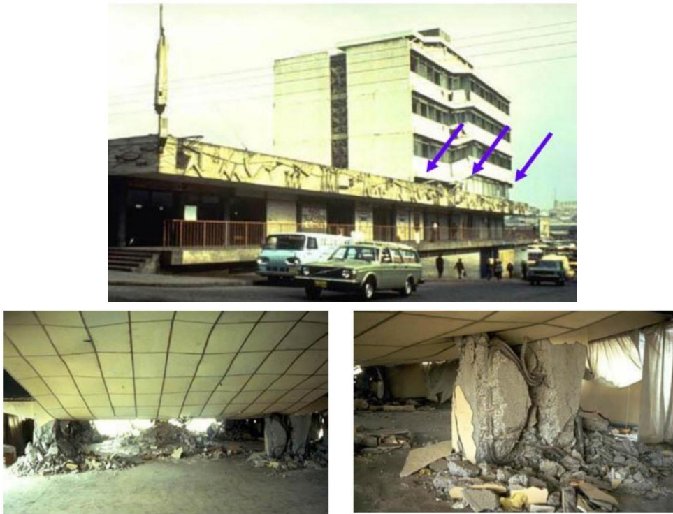
Figure 33 - Damage due to irregularity during Guatemala earthquake 1976, [14]
