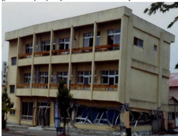
Figure 30 - Damage of three storey building during 1978 Miyagi-Ken-Oki earthquake, [14]
