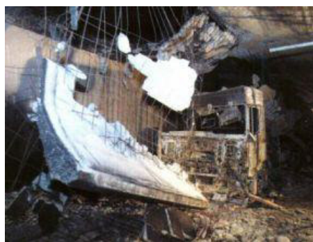
Figure 3. – Collapse of floor construction, exposed to fire [19]
