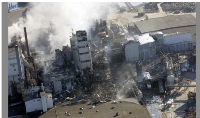
Figure 2 – Imperial Sugar Refinery after explosion in February 2008, Savannah, Georgia, the USA [7]
