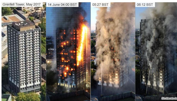
Fig 2. Fire in Grenfell Tower, a west London residential tower block in June 2017 [6]
