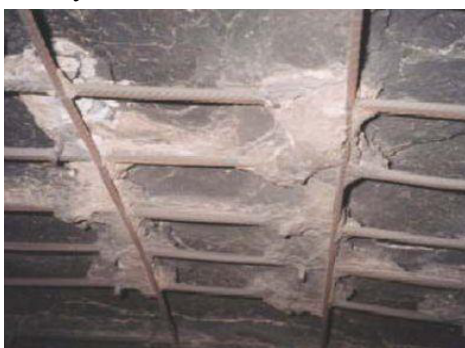
Figure 2. – Separation of the surface overburned layer exposed to fire [2]
