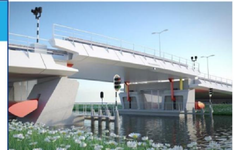
Nelson Mandela Bridge in Alkmaar (NL) FRP movable deck
