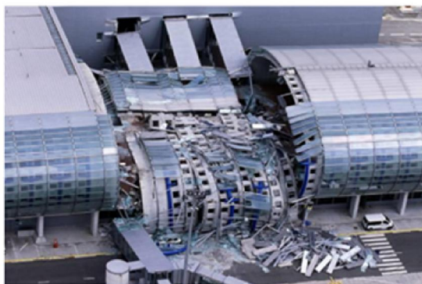
CDG Airport collapse of terminal 2E Paris (2004)
