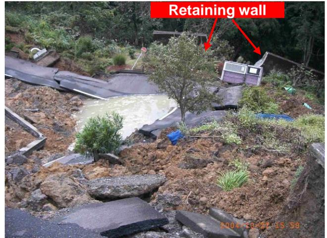
**Photo 2-5 & 2-6.** This residential area was located on small hill terrace. A ring road at the edge of this terrace was wiped off by the landslides on several places. The landslide mass scarped the surface layer just at the edge of the houses, left photo. The right photo also showed retaining wall which was destroyed by landslide.
