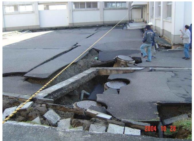
**Photo 4-8** Asphalt pavements and embedded pipe lines were heavily damaged due to ground deformation. Place: N6
