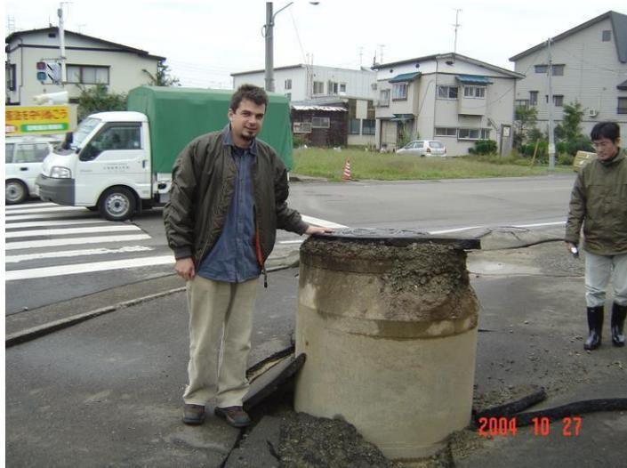
Fig. 3.8 A manhole uplifted during the 2004 Mid Niigata Earthquake
