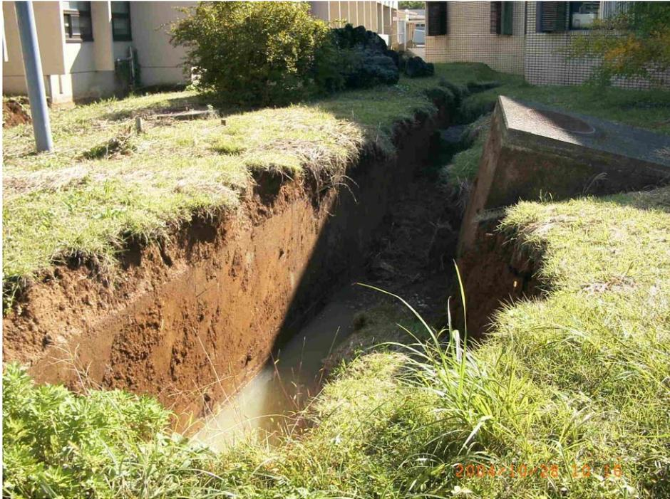
**Photo 4-4.** Fill material separated from underground concrete structure due to large permanent soil displacement. Place : N3, see Photo 4-1
