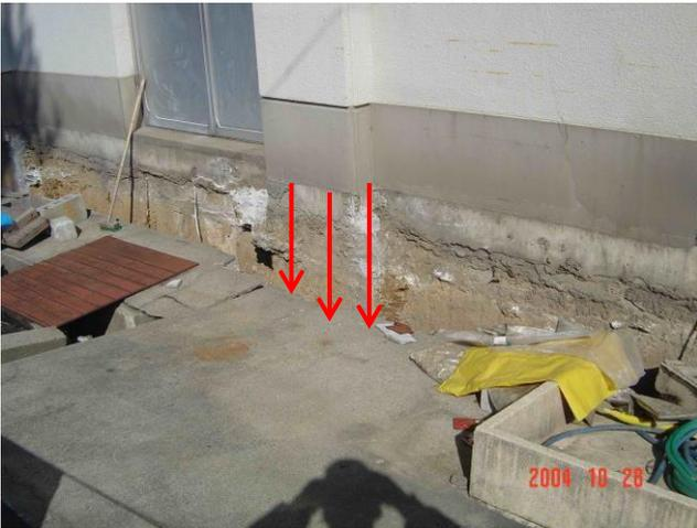
**Photo 4-9.** Soil settlements up to one meter were observed near to this three stories building which is founded on pile foundation. Place: N7
