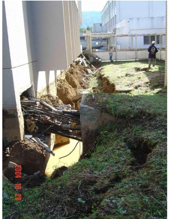
**Photo 4-5 & 4-6.** Large ground deformation was observed between two buildings. RC building which is shown at the left side of the Photos, lay on pile foundation and we didn't observed any significant visual damages. Surrounding soil was completely deformed with large soil displacement and settlements heavily damaging the embedded pipe lines. Place: N4
