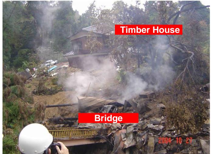
Photos 2-1 & 2-2. Large landslide took place destroying retaining wall and several houses. Soil mass moved more than 50 meters downwards. Place: Nigorisawa
