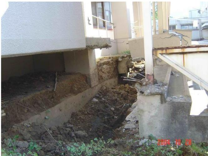
**Photo 4-7** Stairs which lead to entrance of the building (Photo 2-17) were break apart and separated from the building. Place: N5
