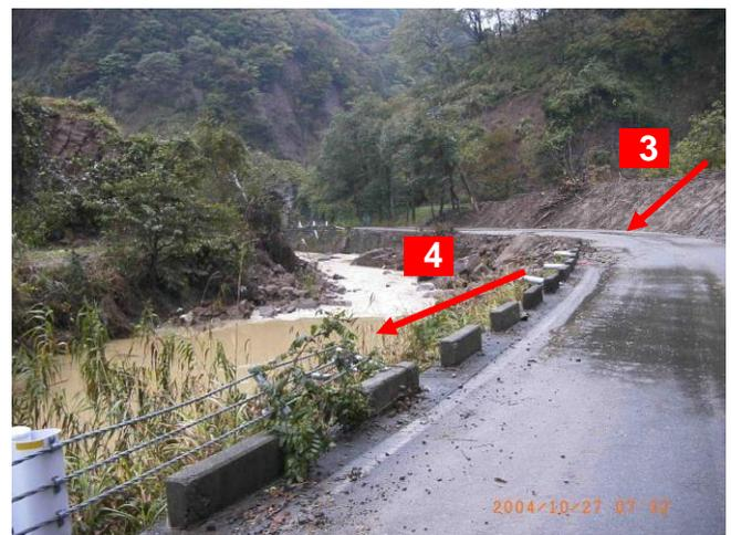
**Photos 1-2 & 1-3** Middle sized landslide in natural slope occurred at this place and temporary blocked the local road and small river. Numbers indicate the steps of the soil movements
