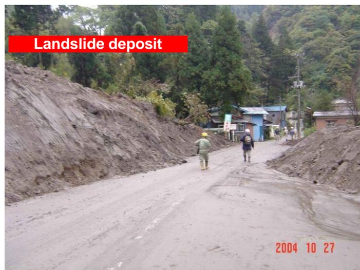
**Photo 1- 4.** Landslide mass temporary blocked the local road, emergency measures had been taken, landslide mass was removed from the road and traffic was enabled again. Place: Nigorisawa
