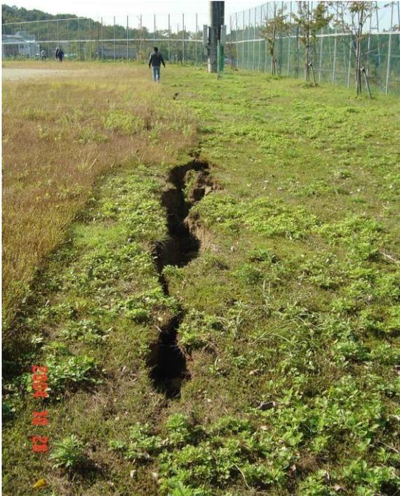
**Photo 4-2.** Soil moved toward the slope of the hill terrace and large cracks appeared at the ground surface. Place: N1, see Photo 4-1.
