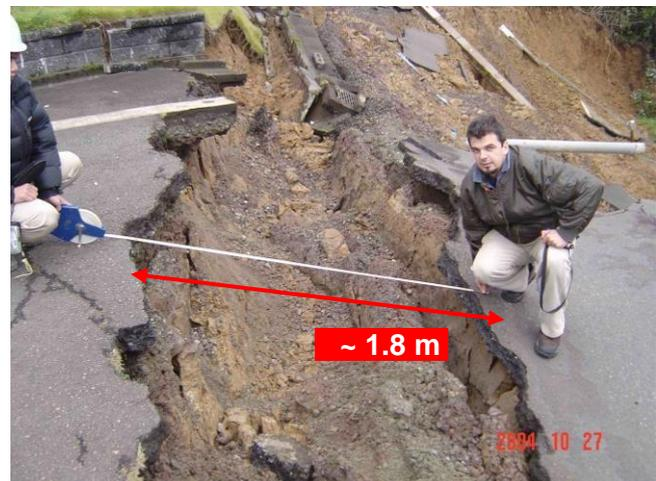
Photo 2-3 & 2-4 Several landslides took place in Takamachi residential area. Large cracks were formed due to soil movement within this area, varied from tens of centimeters to more than one meter. Roads and pipe lines were heavily damaged.
