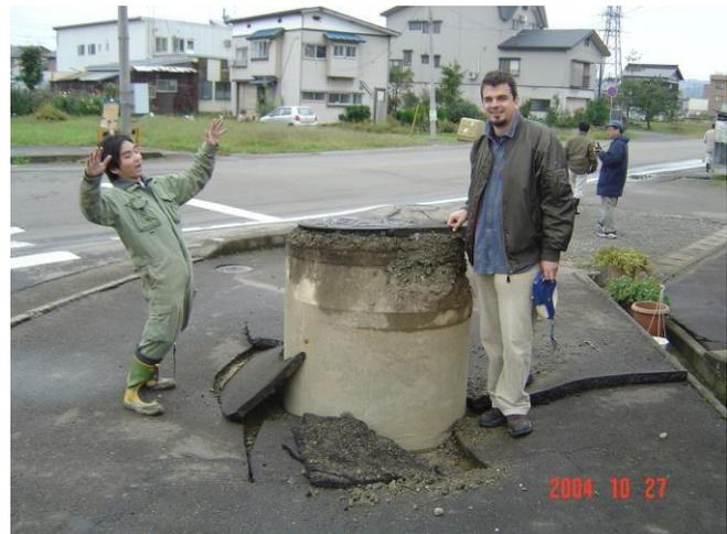
**Photo 3-1 & 3-2** Manhole uplifted by buoyancy force due to liquefaction. Sand ejected from the ground was observed in the vicinity of the manhole
