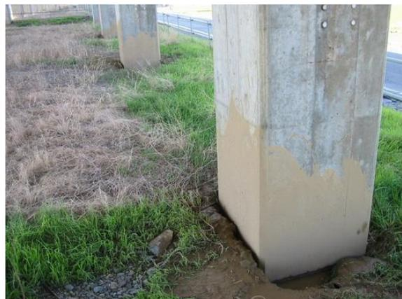
**Photo 3-6** Open gap between pier and ground
