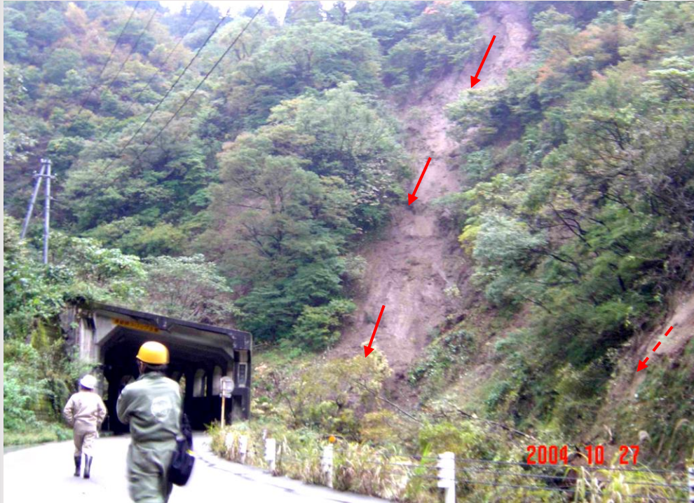
Landslide in steep natural slope
