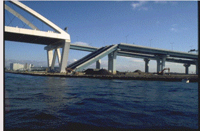
Nishihomiya Bridge - Kobe, Japan
