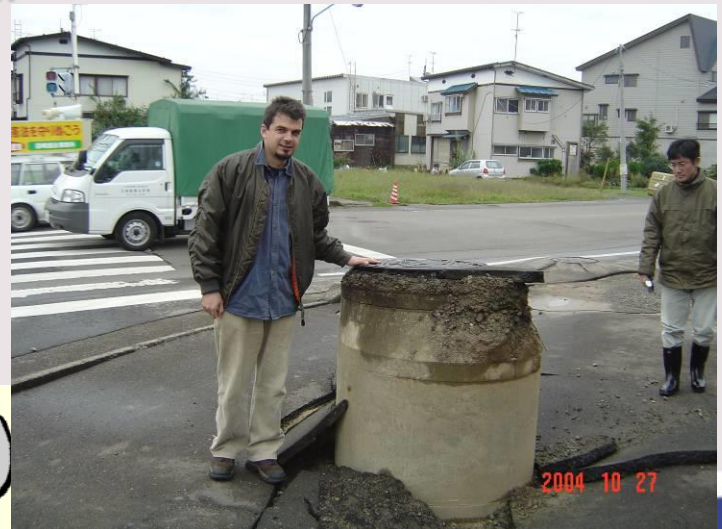
A manhole uplifted during the 2004 Mid Niigata Earthquake
