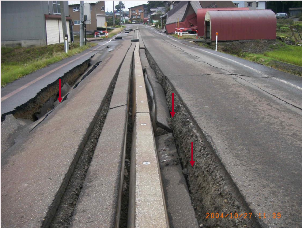
Cracks and subsidence of asphalt pavement.
