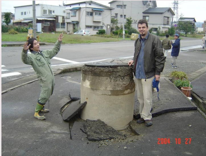
Up-lifted manholes in Ojiya city and small sand boils
