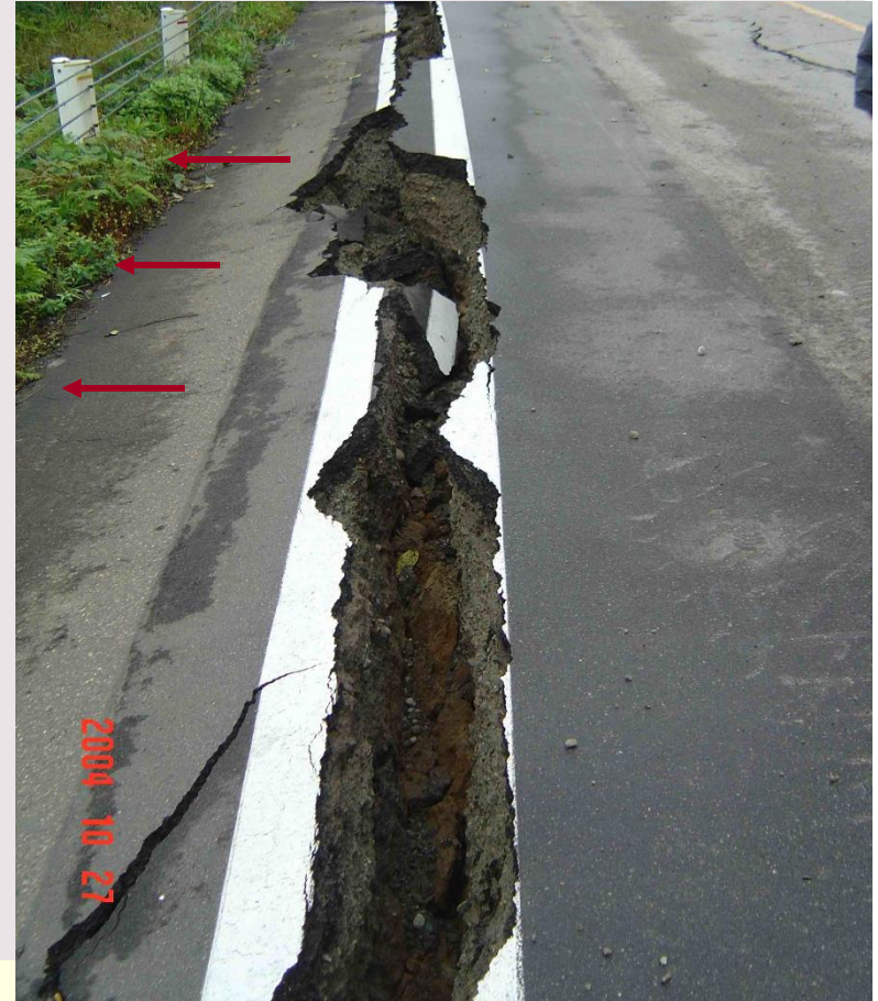
cracks in asphalt pavement due to lateral displacement
