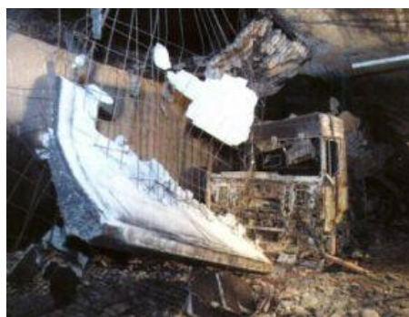
Figure 3. – Collapse of floor construction, exposed to fire [19]
