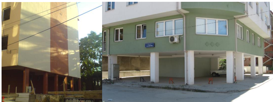
Figure 1 – Reinforced concrete buildings with open first floor
