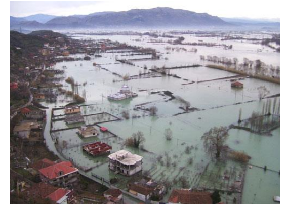
Flooding (public gathering space)
