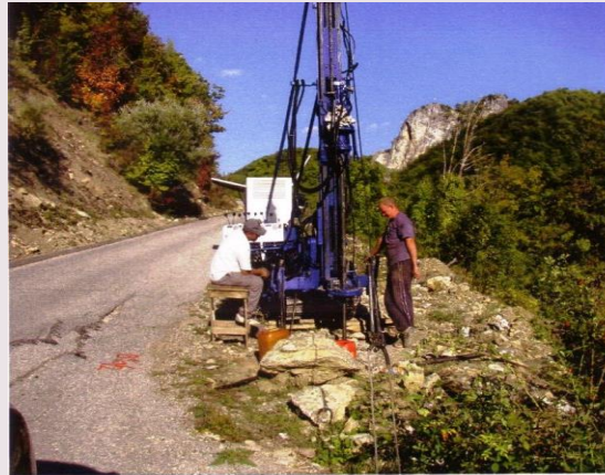
Probe drilling with sampling
