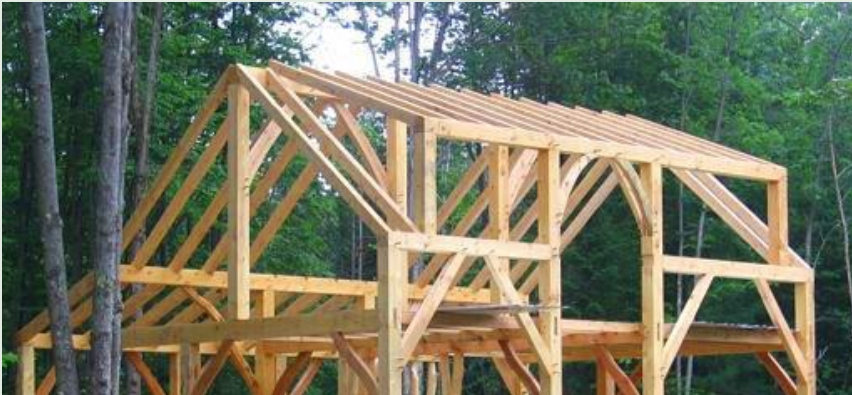
Traditional house - Timber frame structure
