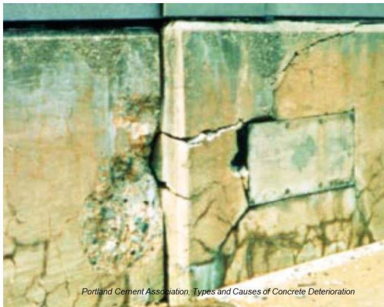
Figure 14– Alkali-silica reaction in concrete
