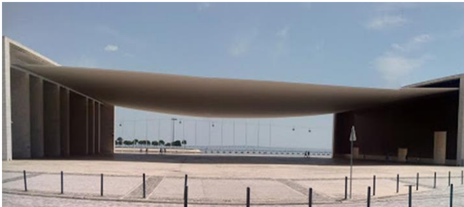
Figure 1 – Giant prestressed concrete slab, Portuguese National Pavilion, Lisbon
