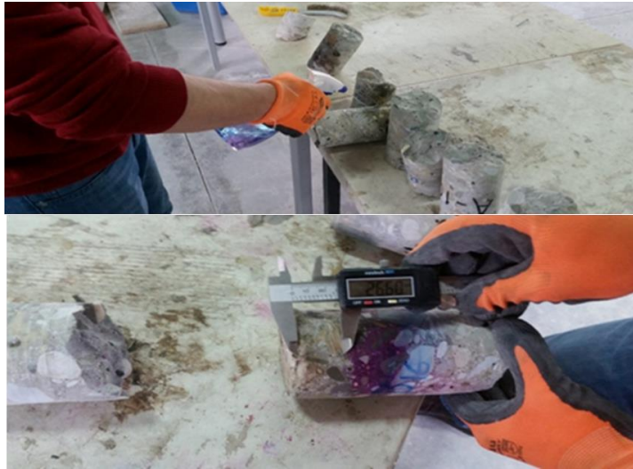
Figure 15– Measuring of carbonation depth with Phenolphthalein solution
