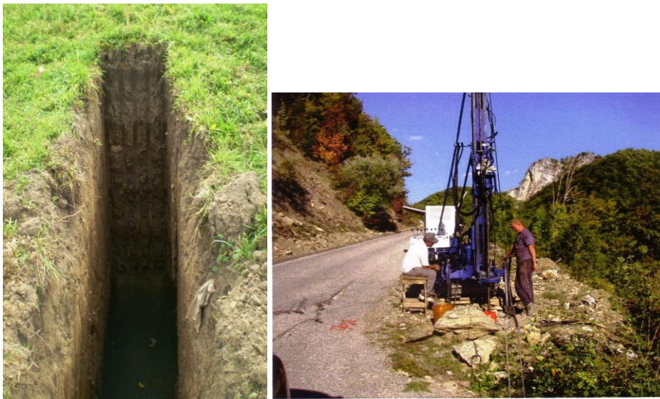
Figure 13. Probe ditch for sampling (left) and Probe drilling with sampling (right).
