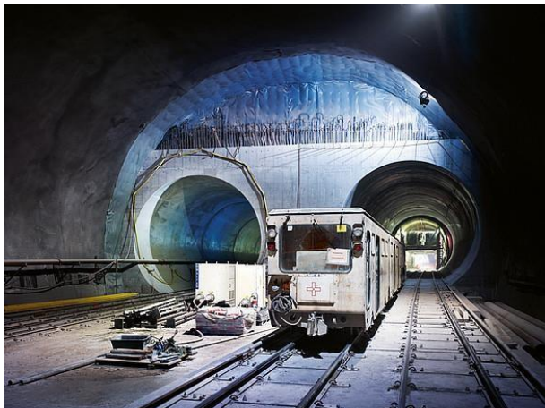
Figure 1 – Gotthard Base Tunnel – Switzerland (The longest and deepest railway tunnel in the world, L = 57 km (single tube), H = 2,45 km (maximum depth))
