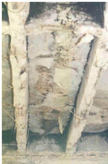
Fig. 19. Influence of defects on fire damages degree in pan joist floor system
