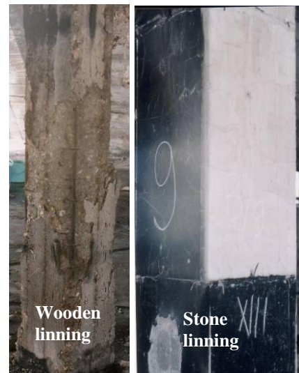
Fig. 20. Influence of type of decorative layer type on the fire damage degree of concrete columns
