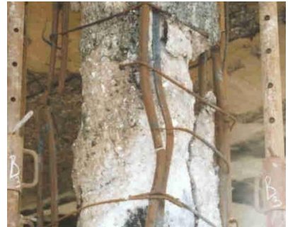
Figure 8: Plastic deformations and breaking off of bars
