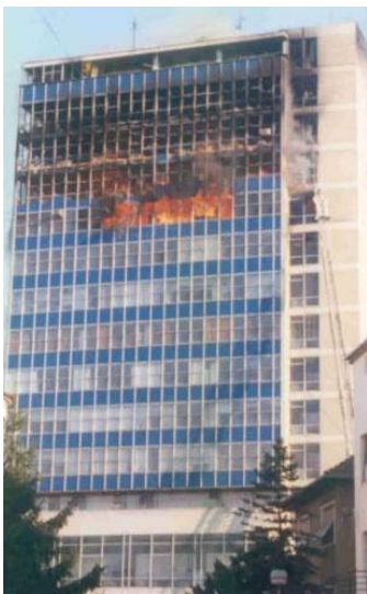
Fig. 18. Spreading of fire in both vertical directions [9]
