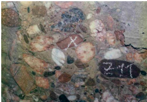
Figure 1: Aggregate spalling
