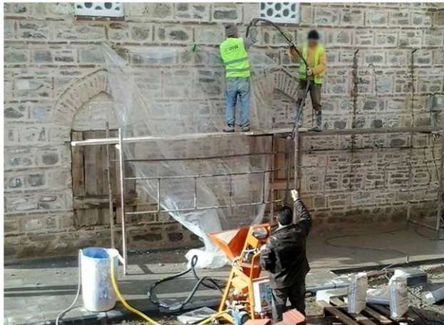
Figure 6 - Application of injection mix [24].
