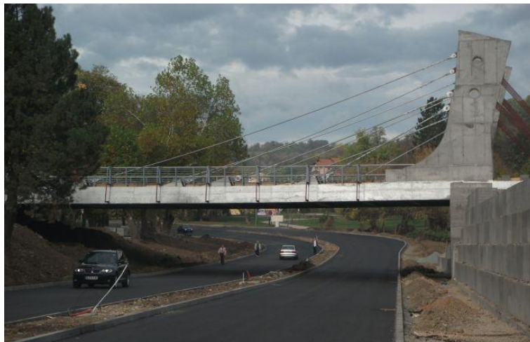
Figure 9 - View of the bridge
