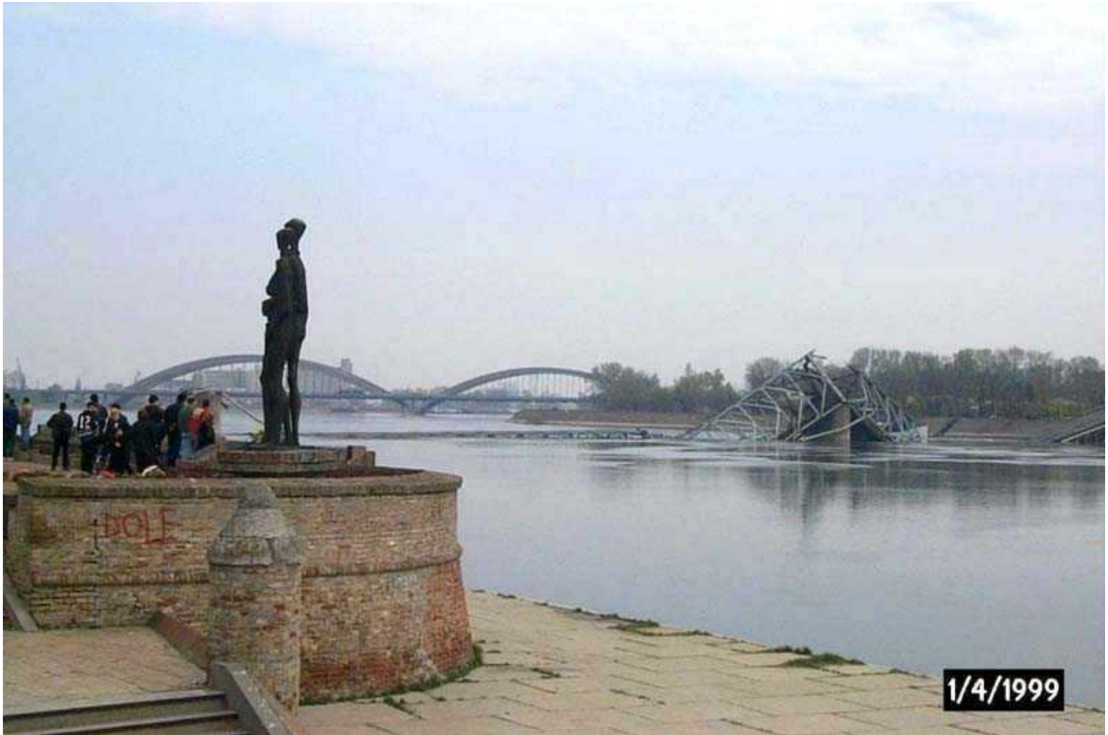
Ruins of Varadin Bridge
