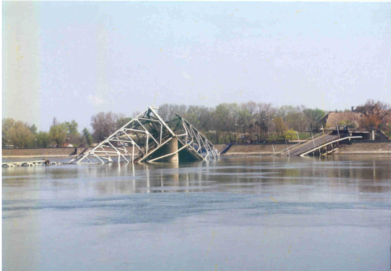
Ruins of Varadin Bridge over the River Pier on Petrovaradin Side
