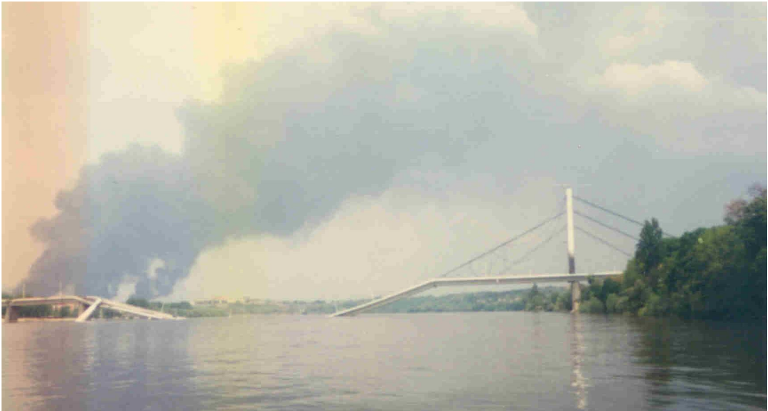
Broken Main Span and Pylon
