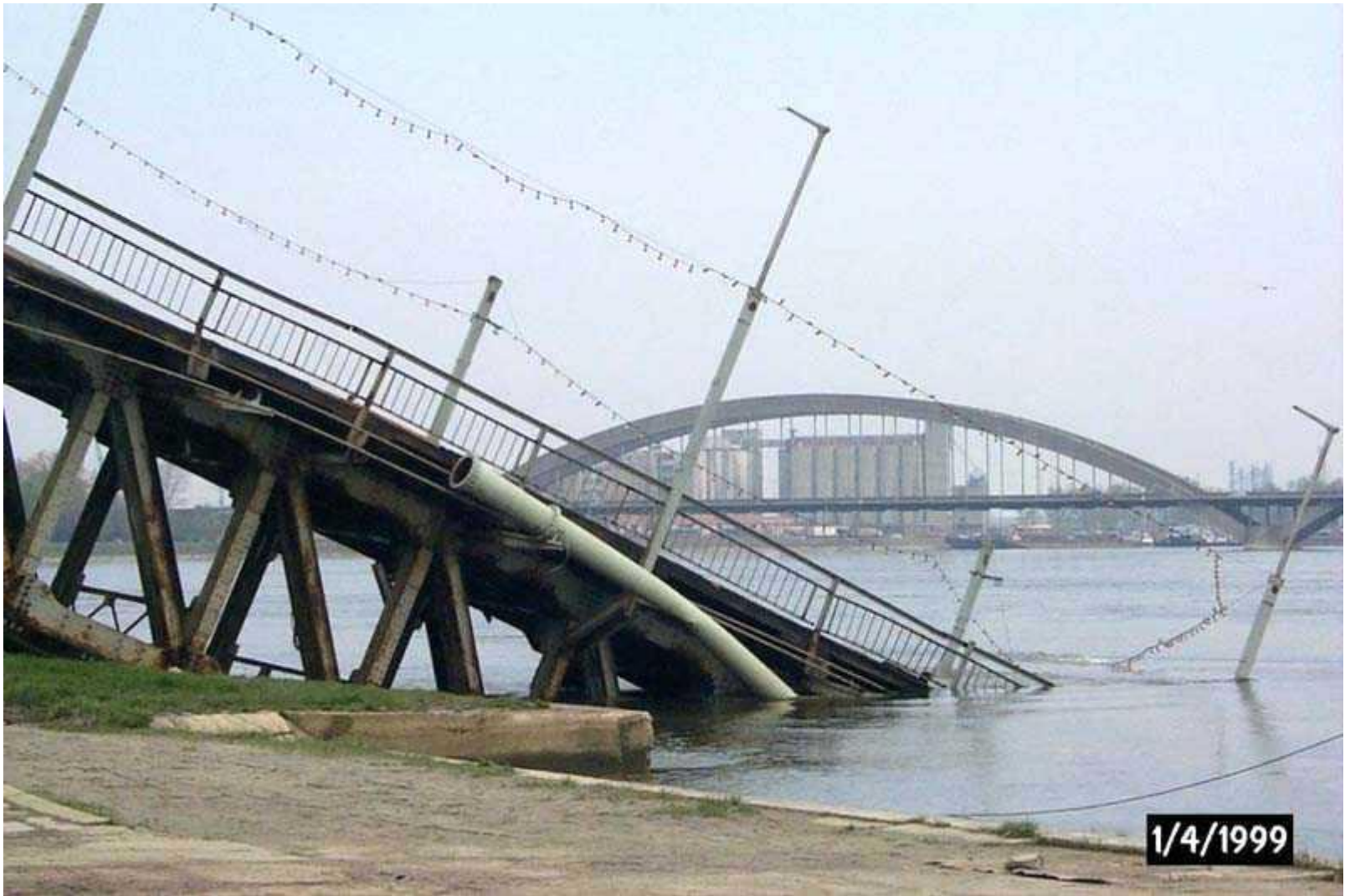
Ruins of the Inundation Structure of Varadin Bridge on Novi Sad Side
