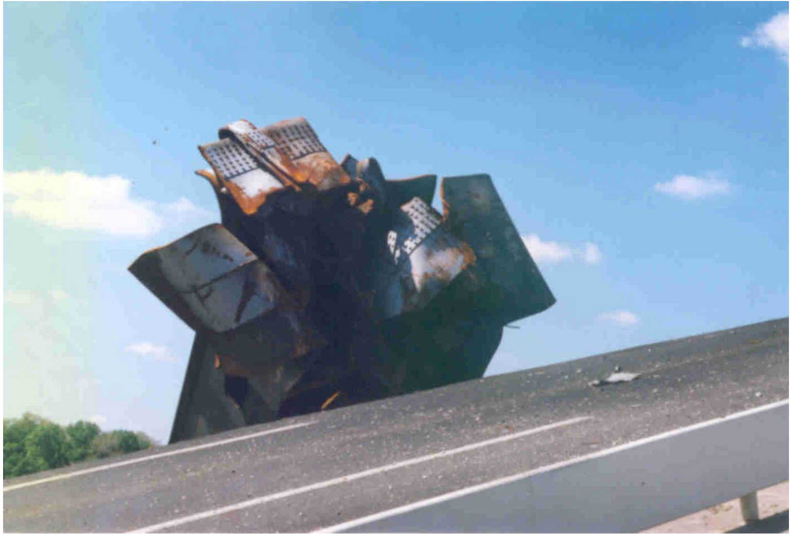
The Sight of the Destroyed Pylon
